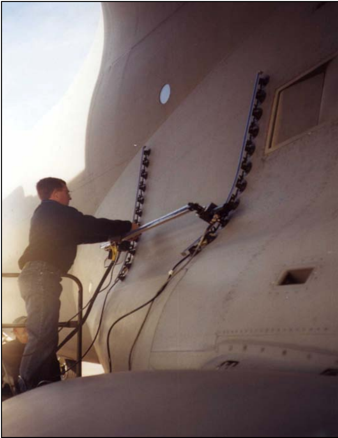
Catamaran scanner being installed on the fuselage of a C-17 aircraft.
